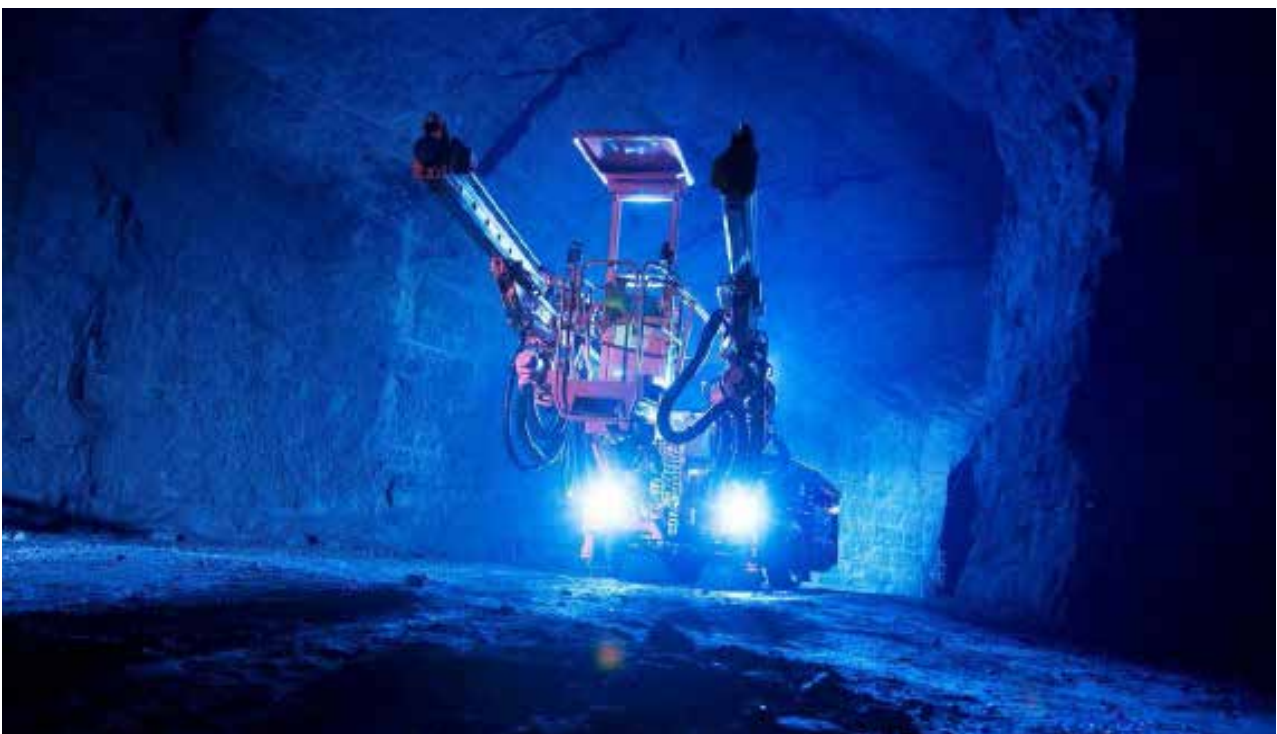
1. SANDVIK DT821 - TUNNELING DRILL
