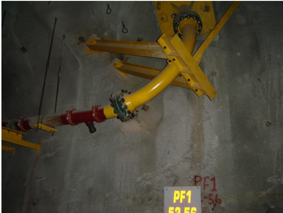
Figure 16.20 – Typical Borehole to Level Piping Connection Configuration
