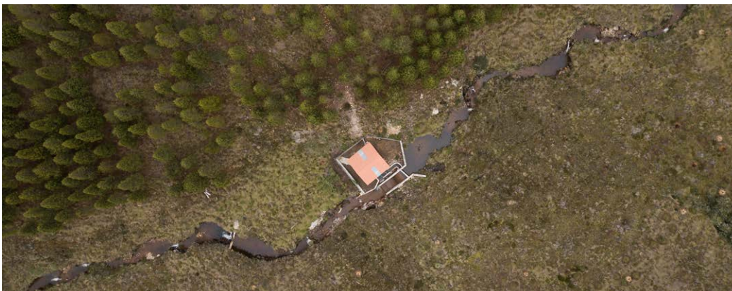
Water monitoring station at our Loma Larga project in Ecuador.
